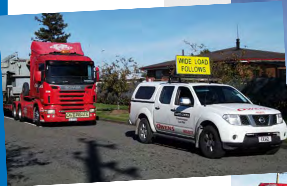
Removing transformers from Bexley Substation to ABB's workshop to be refurbished
